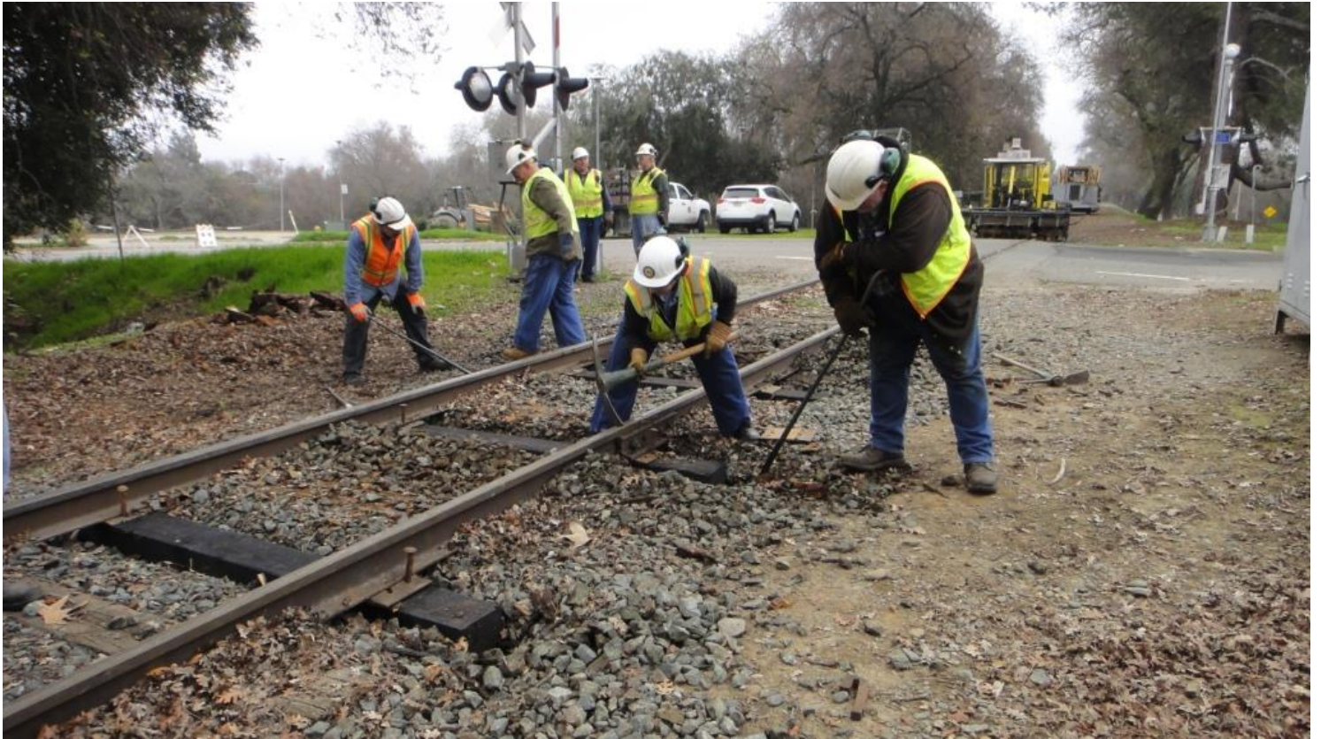
Frank nips-up the new tie while Pam uses the maddox to shove some rock under it for support
