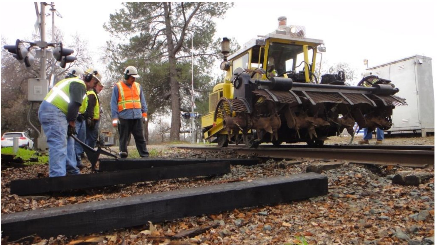
Mike F. guides a new tie into place as Alan in the scarifer uses the inserter function to pull it into the crib
