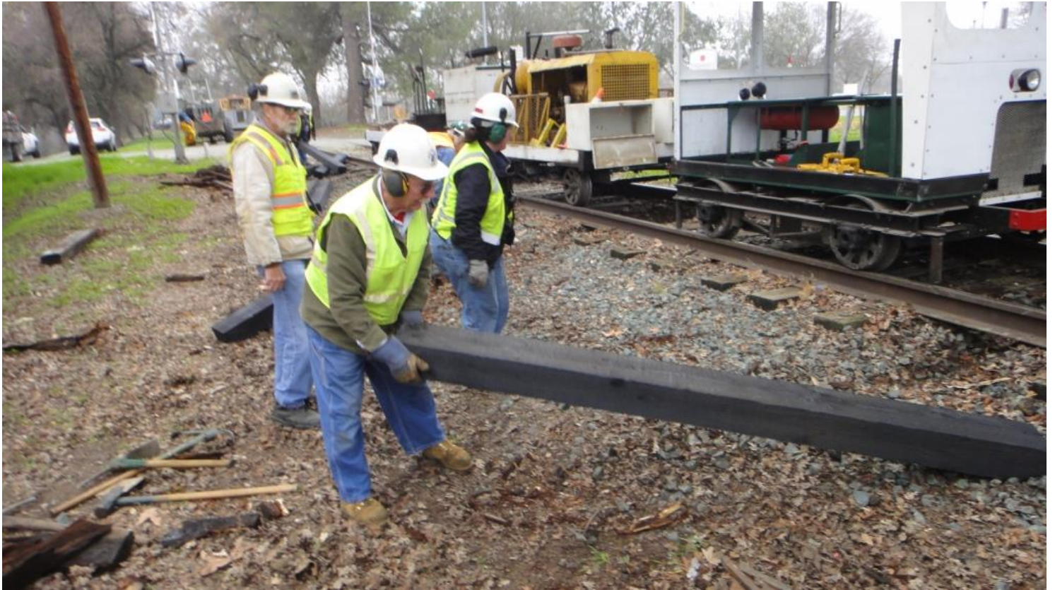
With the old tie removed, Clem spots a new tie for insertion
