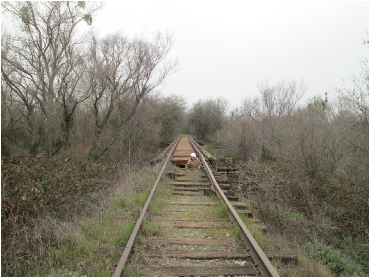
Mike T. inspects the approach to Trestle 4. Yeah, it's a no-go...
