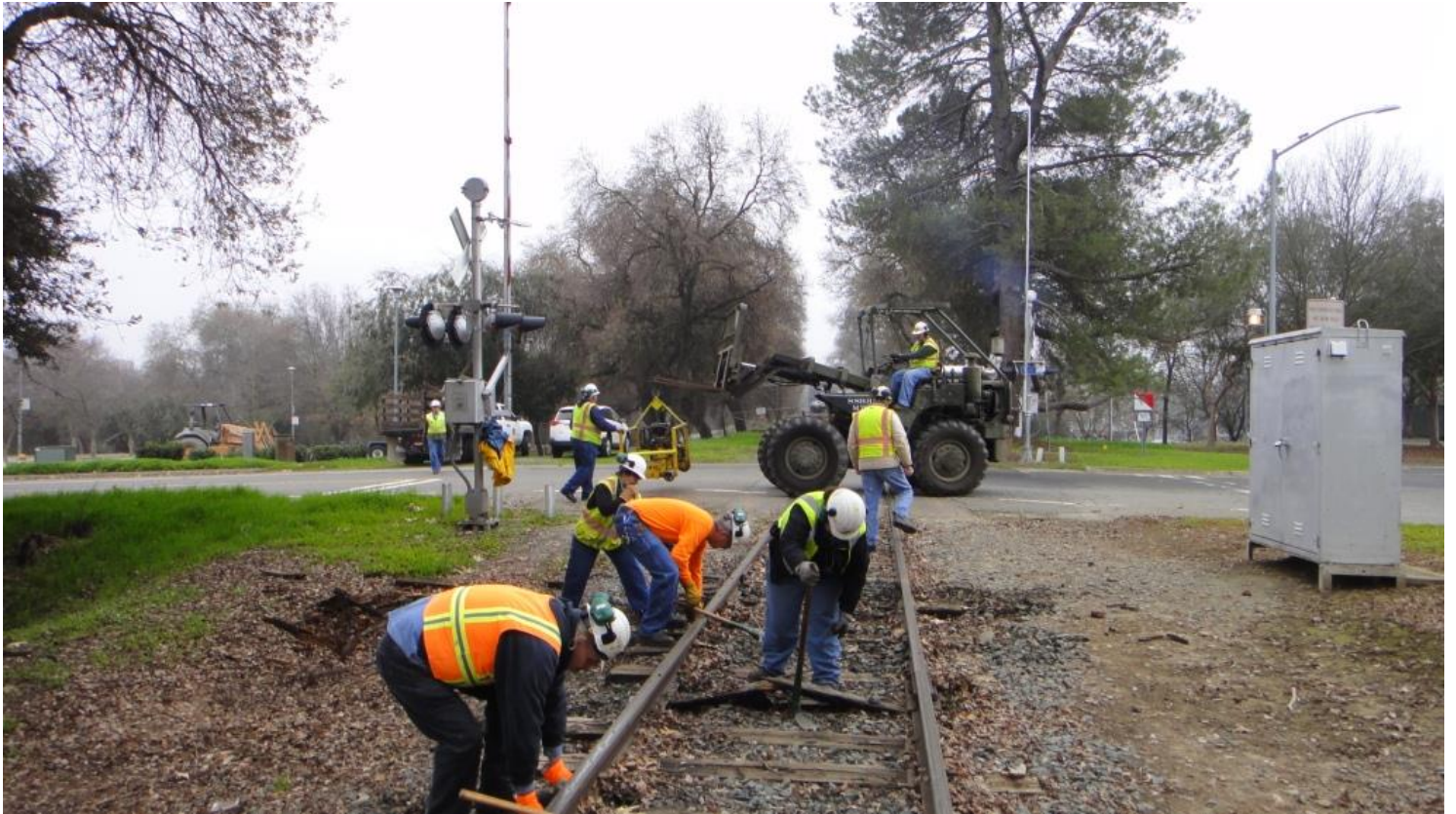
Mike F. on Big Green deploys the section-gang machine while the Team preps the ties for pulling
